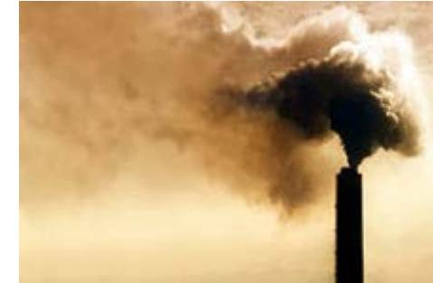
Flue gas cleaning
