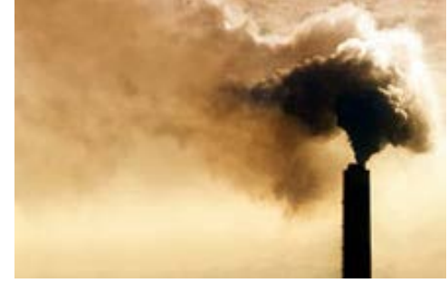
Flue gas cleaning
